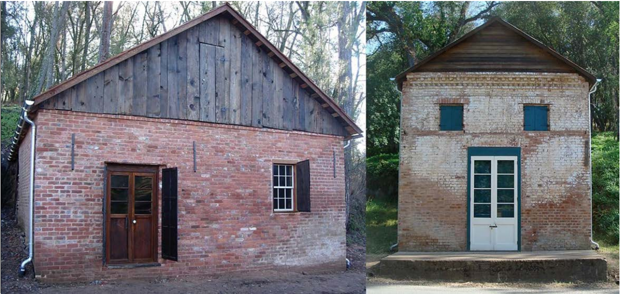
Fiddletown's restored Chinese gambling hall (left) and general store
