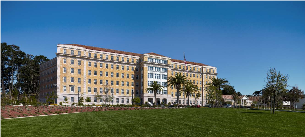
The fully restored Public Health Service Hospital at the Presidio.
