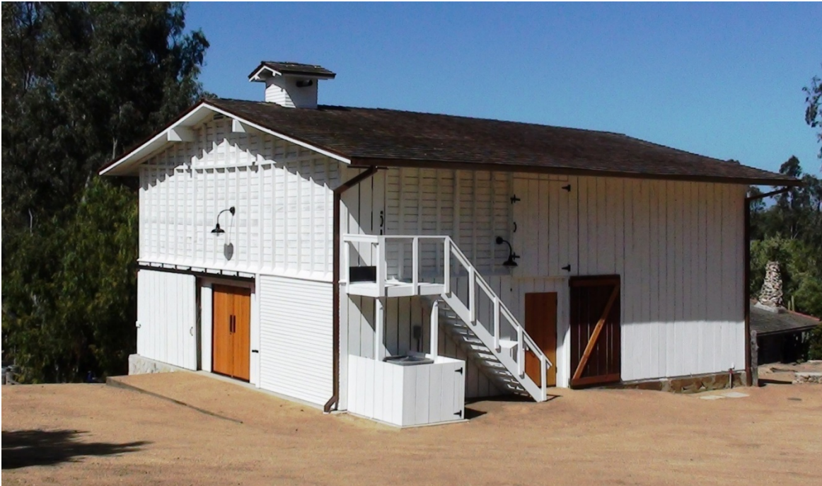
The restored and stabilized Leo Carrillo Ranch Barn
