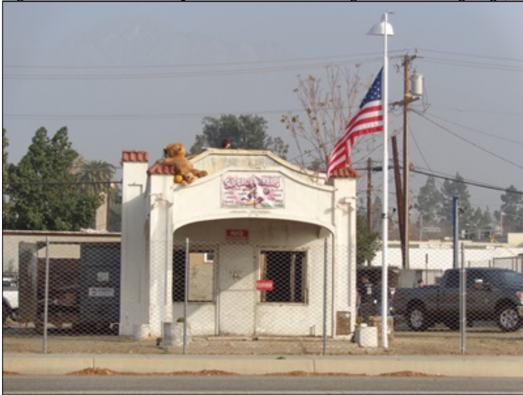
Figure 9: Pre-restoration photo of station following demolition of garage, circa 2013.
