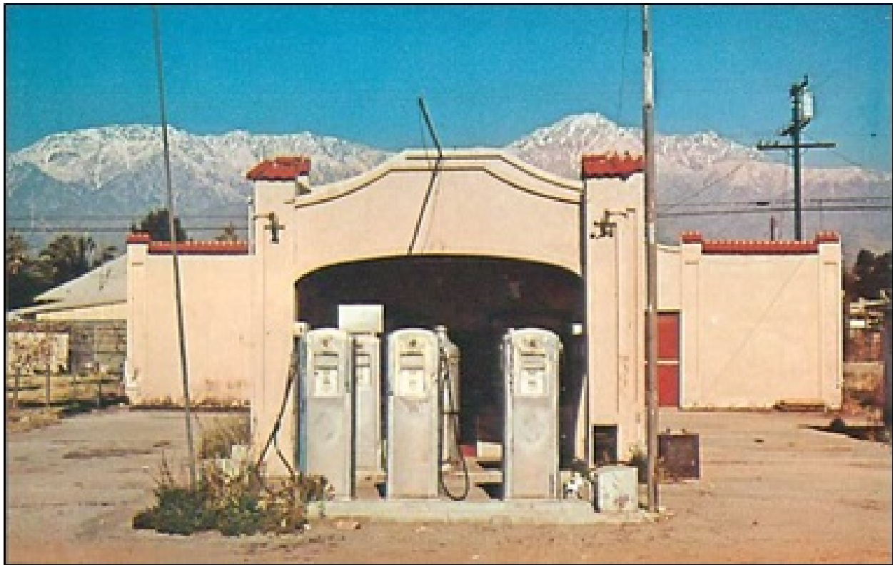
Figure 5: View of station after 1972 business closure.
