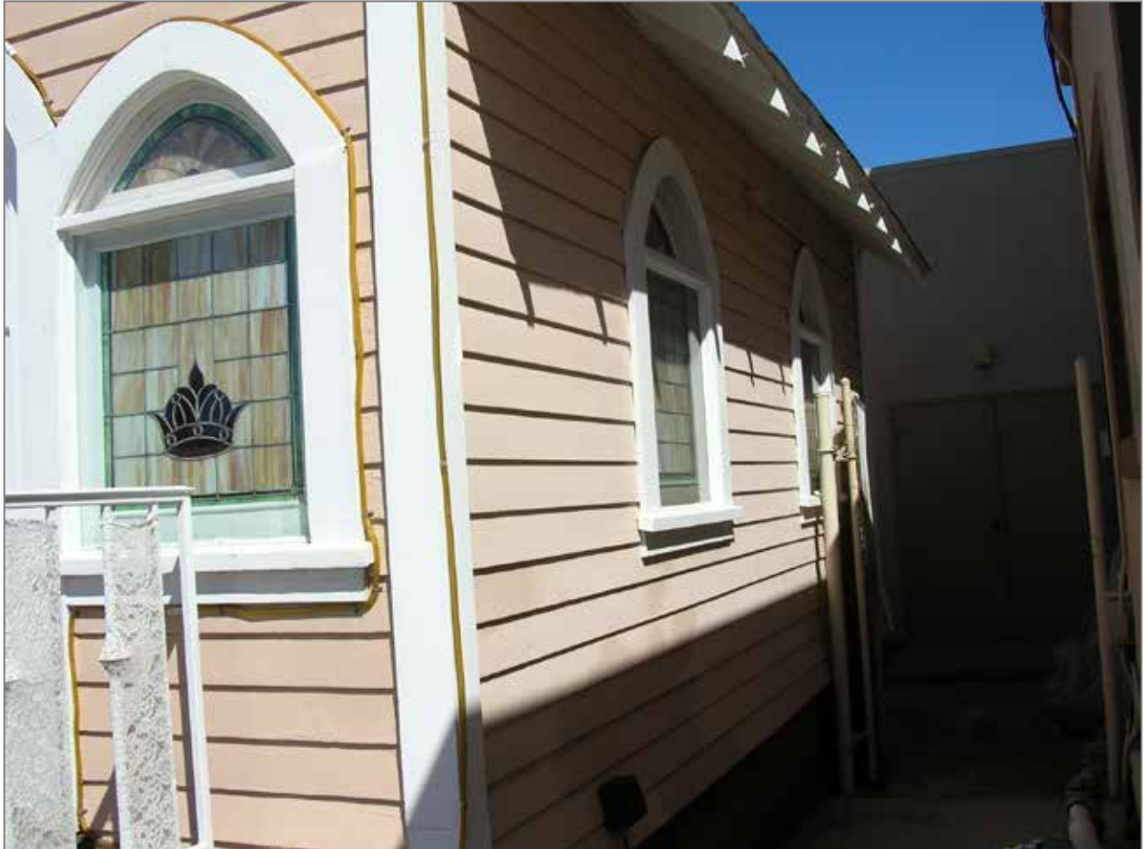
Photo 3: Portuguese Chapel, primary and south side facades (north view)
