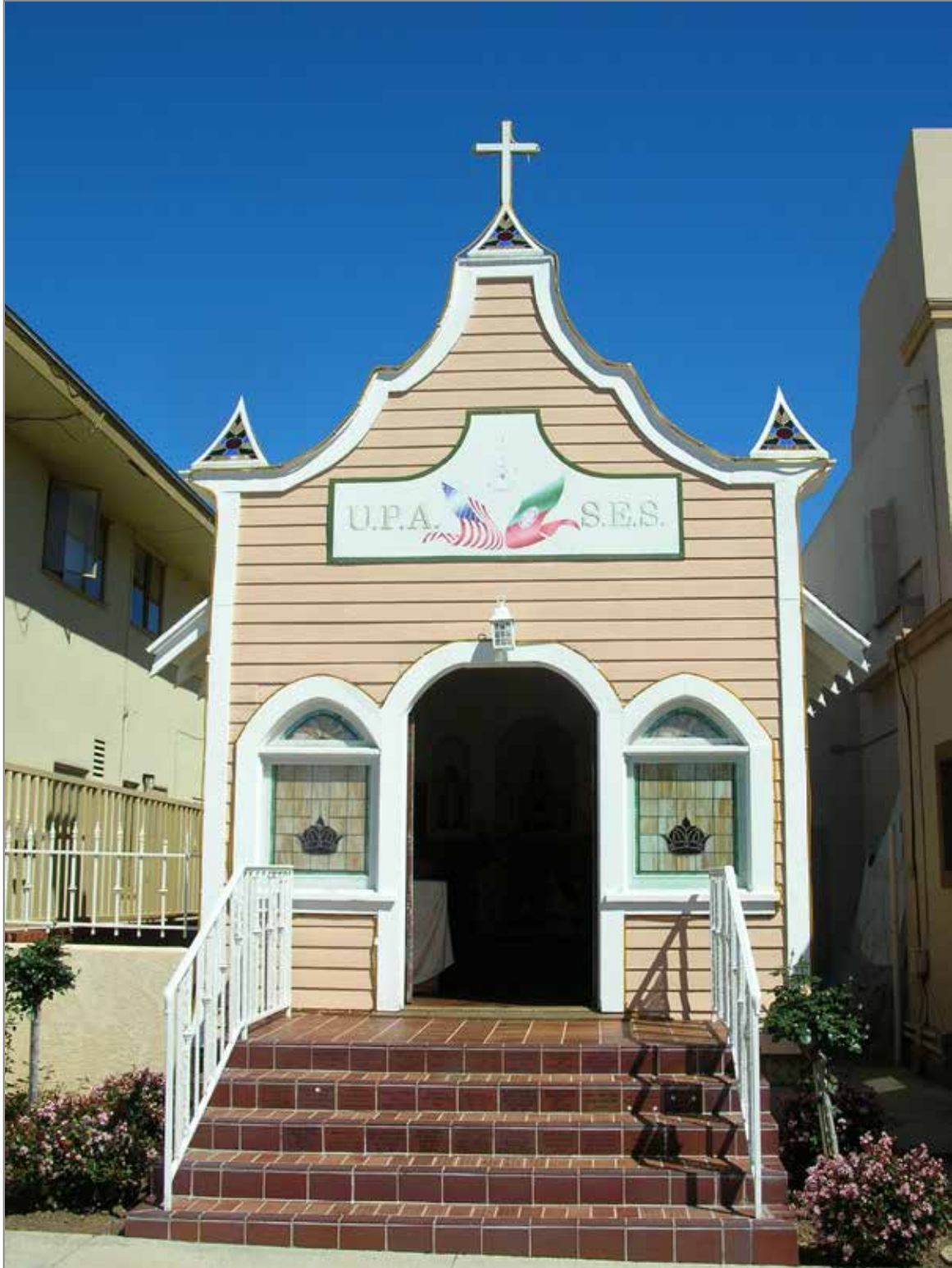
Photo 2: Portuguese Chapel, primary facade (northeast view)
