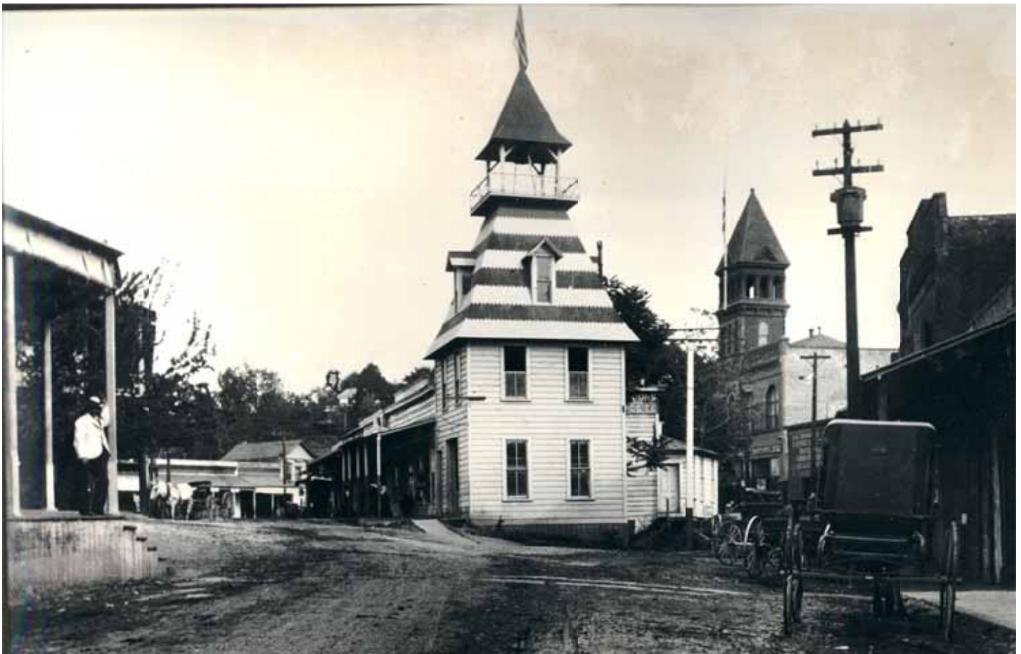
Figure 1 of 4 Historic Fire House No 2 c 1896
