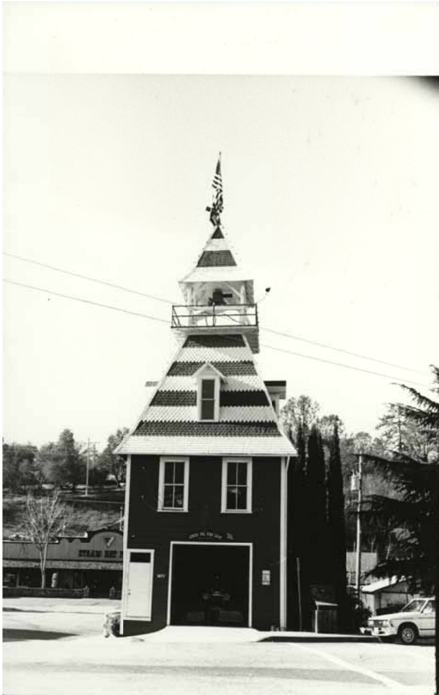
Figure 4 of 4 Historic Fire House No. 2 c 1980
