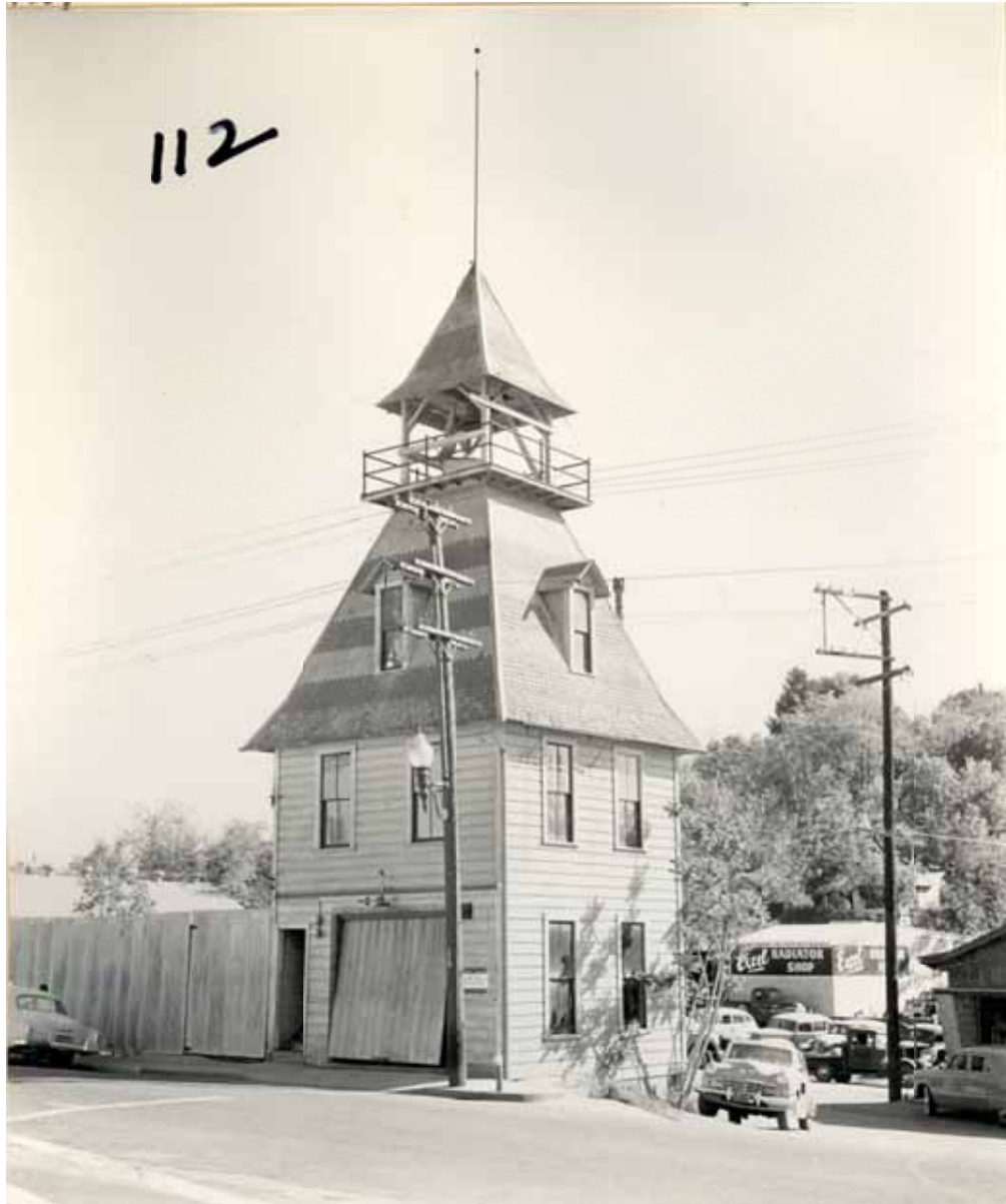
Figure 3 of 4 Historic Fire House No. 2 c.1954
