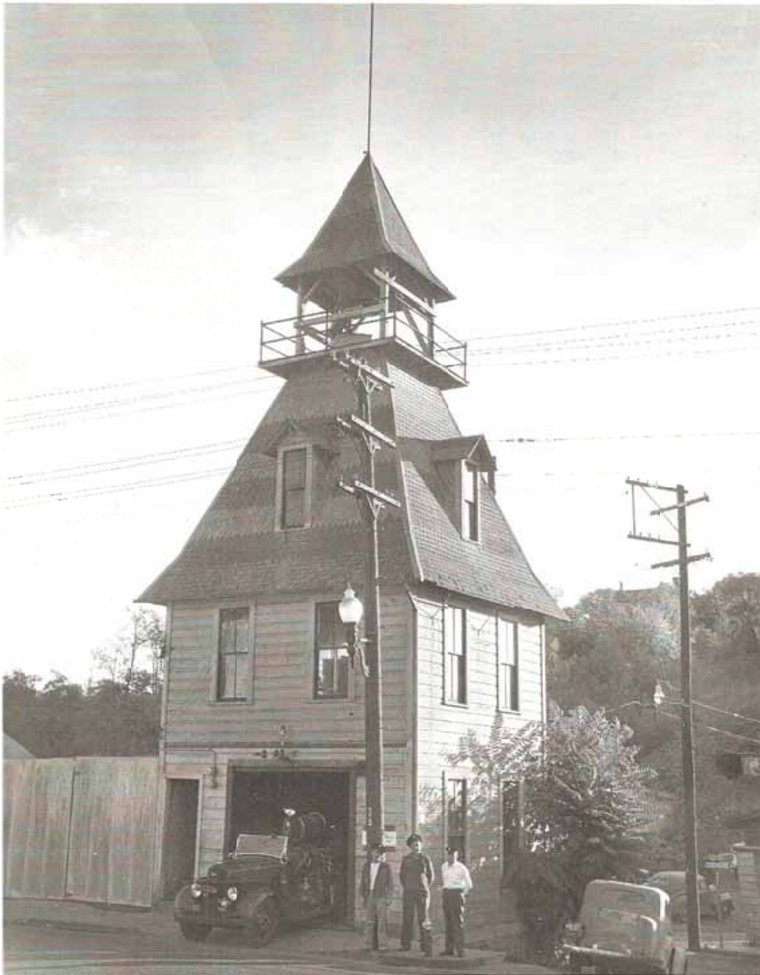
Figure 2 of 4 Historic Fire House No 2 c. 1940
