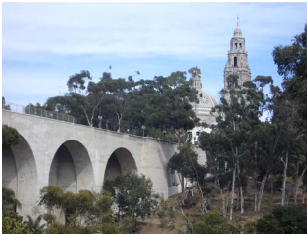
Cabrillo Bridge and Balboa Park
